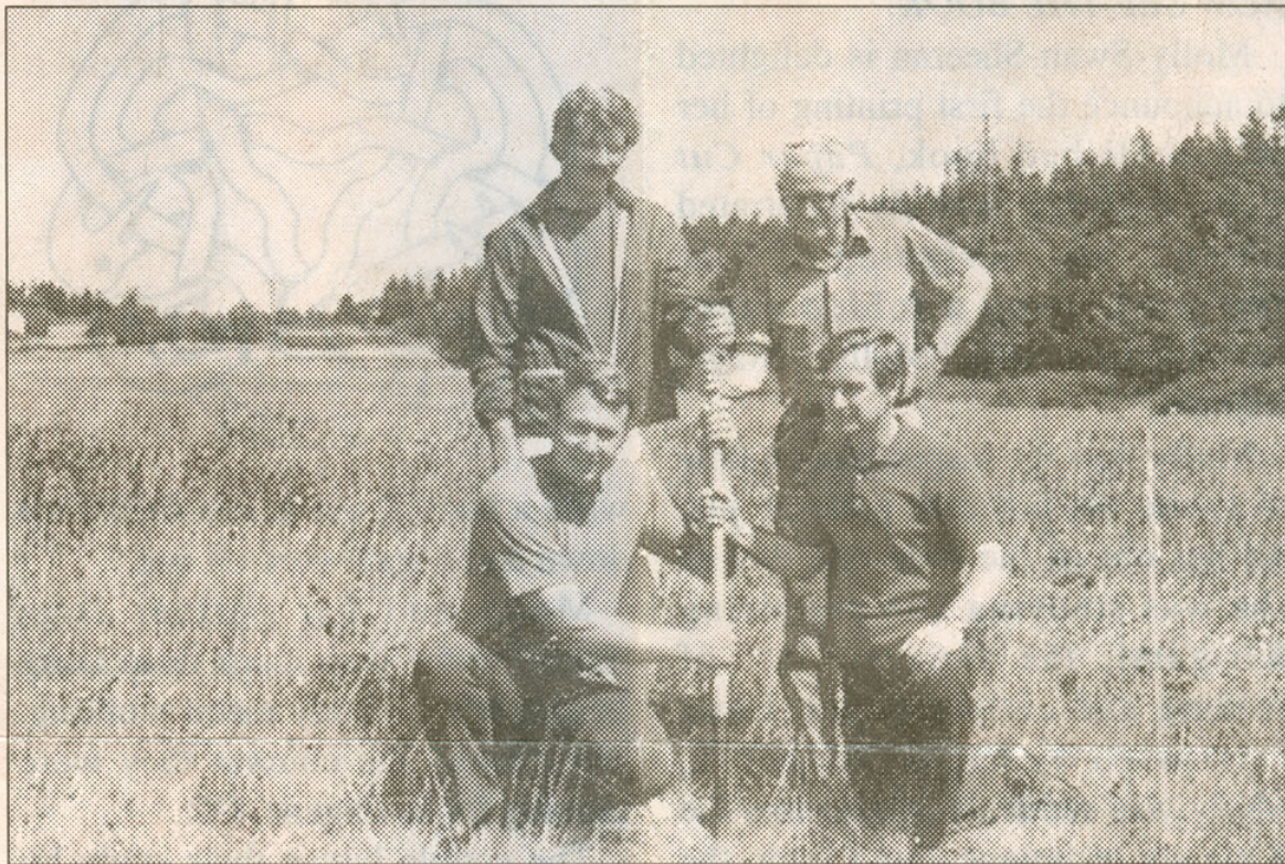
clockwise: Don Poole (contractor), Jerry Eads (original property owner), John Ottenheimer (architect) and Charlie Washburn break ground for the original Lopez Clinic in 1973. It was named after Washburn's wife Catherine.
